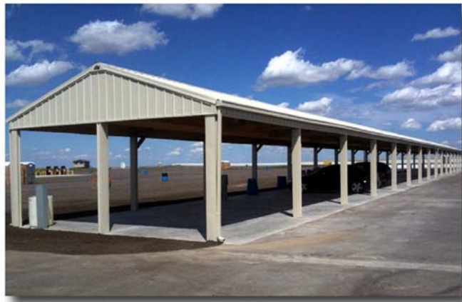
New Carports at HPR
